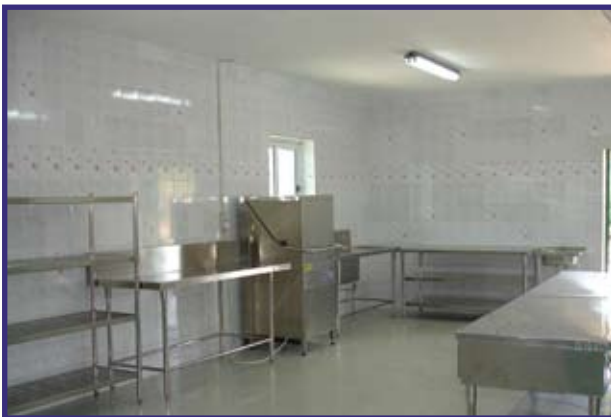
The kitchen inside during the construction
