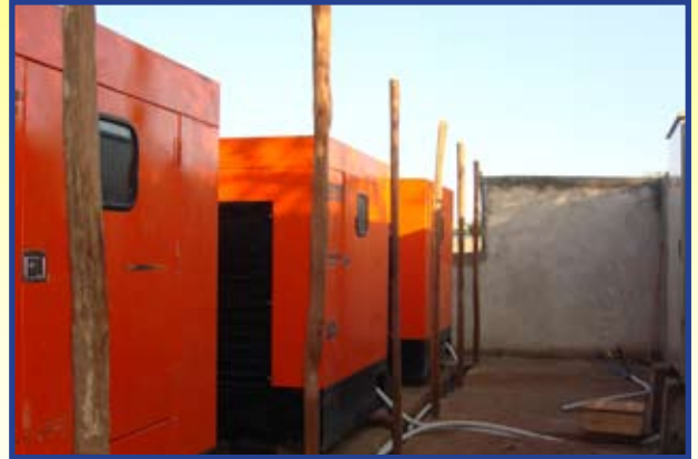
Three generators, each on 400 KVA
