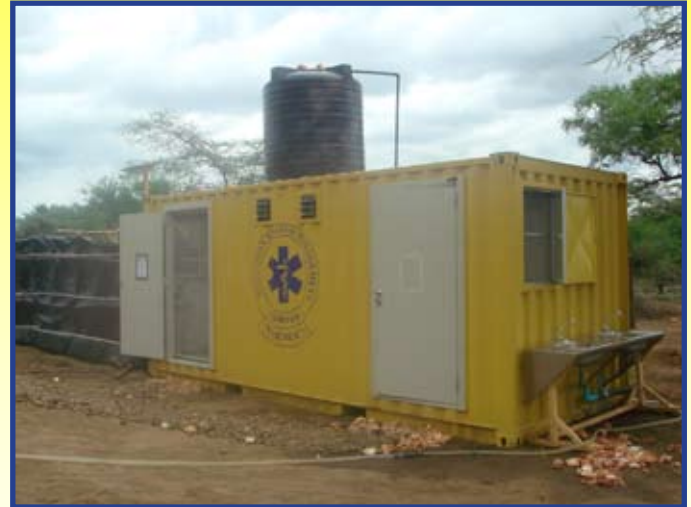
Toilets and shower used during the construction
