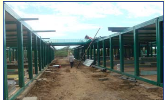
The hospital alone is 162 flatpack containers.
